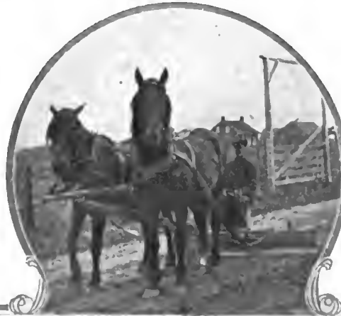
These three illustrations show actual work on the roads of one of our Southern states. The road in this instance was composed of a soft dirt or clay which made an excellent roadbed in dry weather, but which became a morass almost at the first touch of rain. By the use of the drag the community was able to keep the roads in a fairly good condition even in the rainy season. In winter the ruts which froze solid prevented satisfactory touring through this particular section
